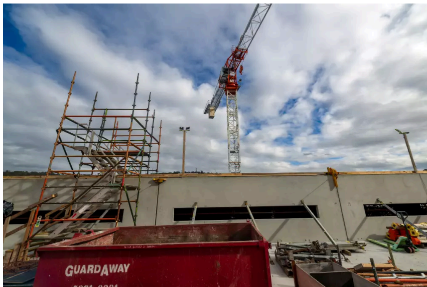
The Launceston Health Hub expansion under construction. Picture by Phillip Biggs
